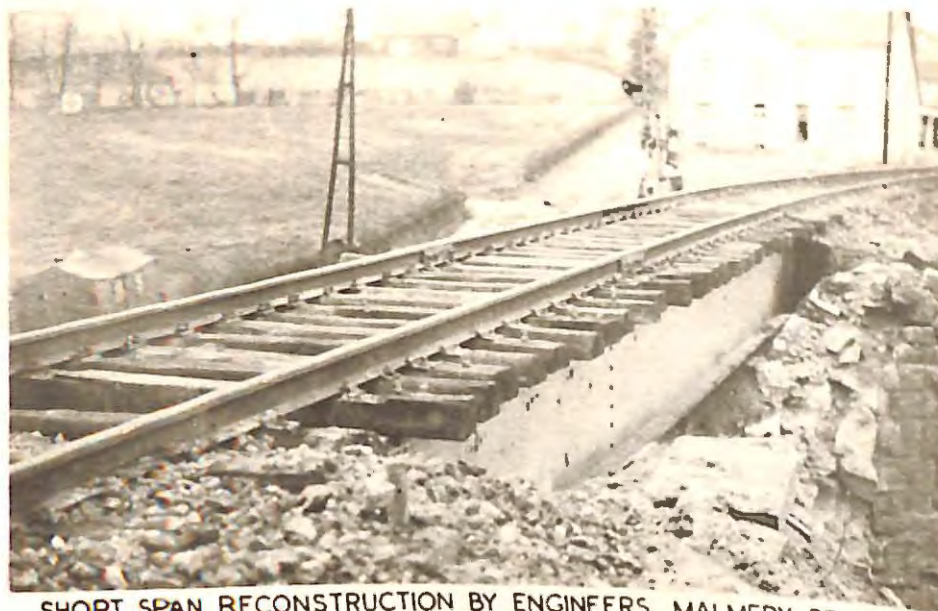
SHORT SPAN RECONSTRUCTION BY ENGINEERS. MALMEDY. BELGIUM
