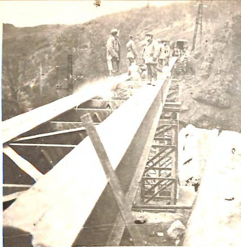
ENGINEER BRIDGE RECONSTRUCTION MALMEDY. BELGIUM
