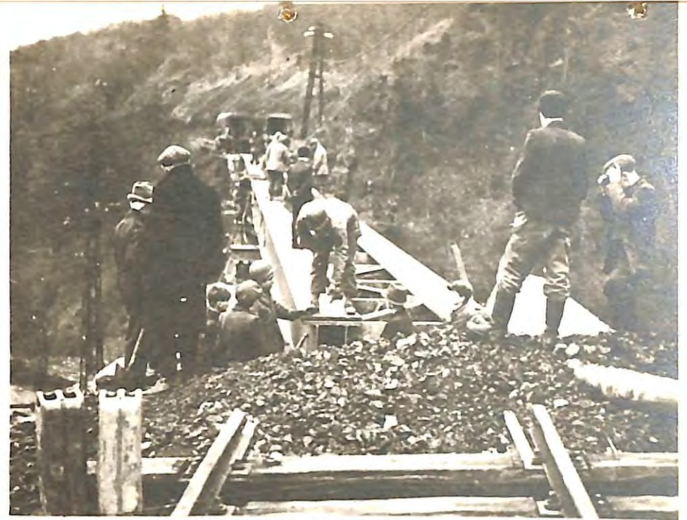
ENGINEER CORPS BRIDGE RECONSTRUCTION - BELGIUM
