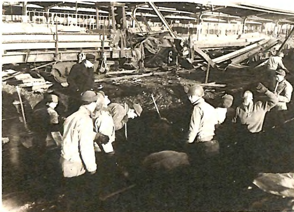
REPAIRING DAMAGE IN RAILYARDS - BELGIUM
